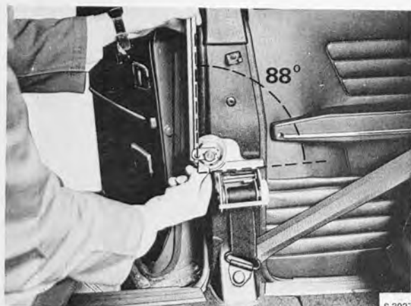
ANGLE BETWEEN RETRACTOR AND REAR EDGE OF DOOR PILLAR CHECKED WITH A GRADUATED ARC
