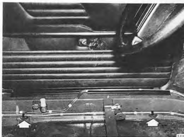
DRAIN HOLES IN THE SILLS
