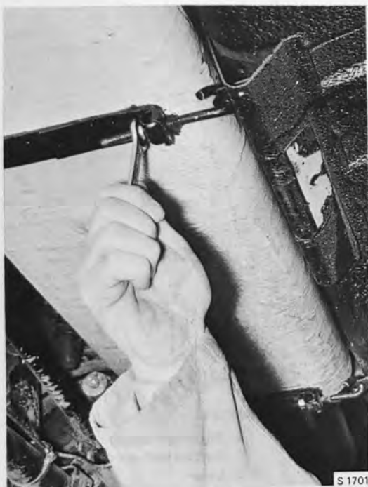
REMOVING THE FUEL TANK
