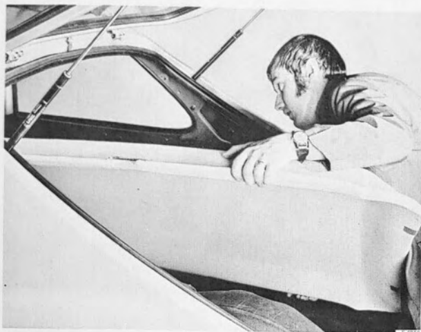
REMOVING THE HEAD LINING
